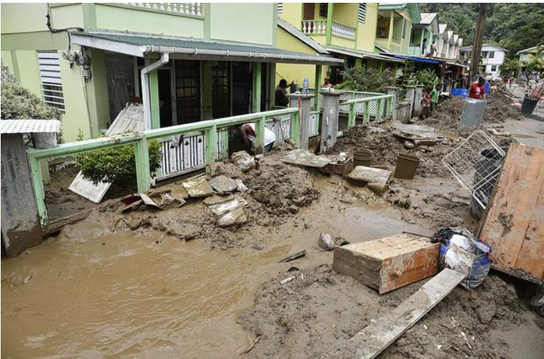
Some of the damage in Bath Estate, one of the nine disaster areas from hurricane Erika 08/26/15 (Photo courtesy Government of Dominica)
